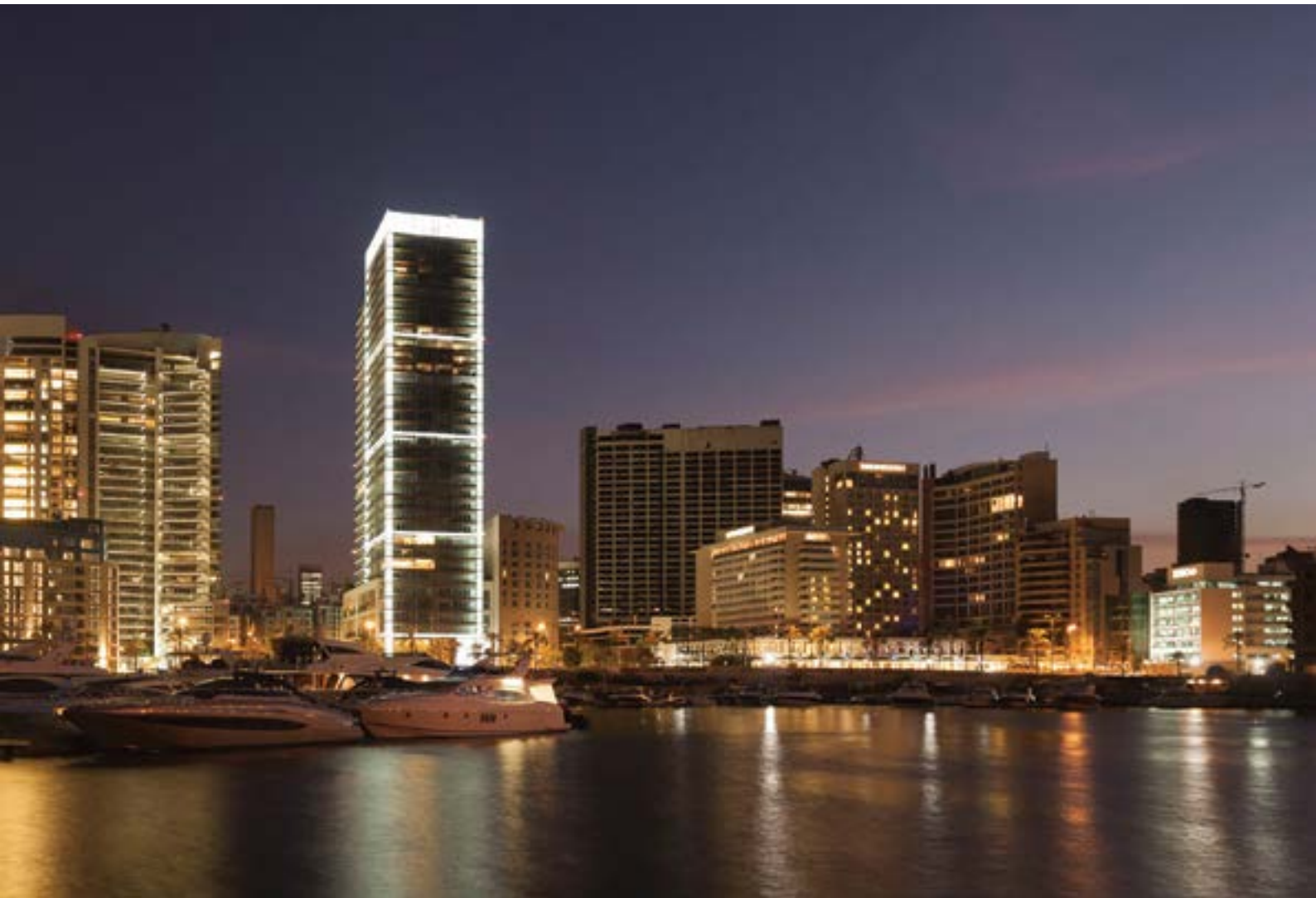
Platinum Tower, Beirut, Lebanon
