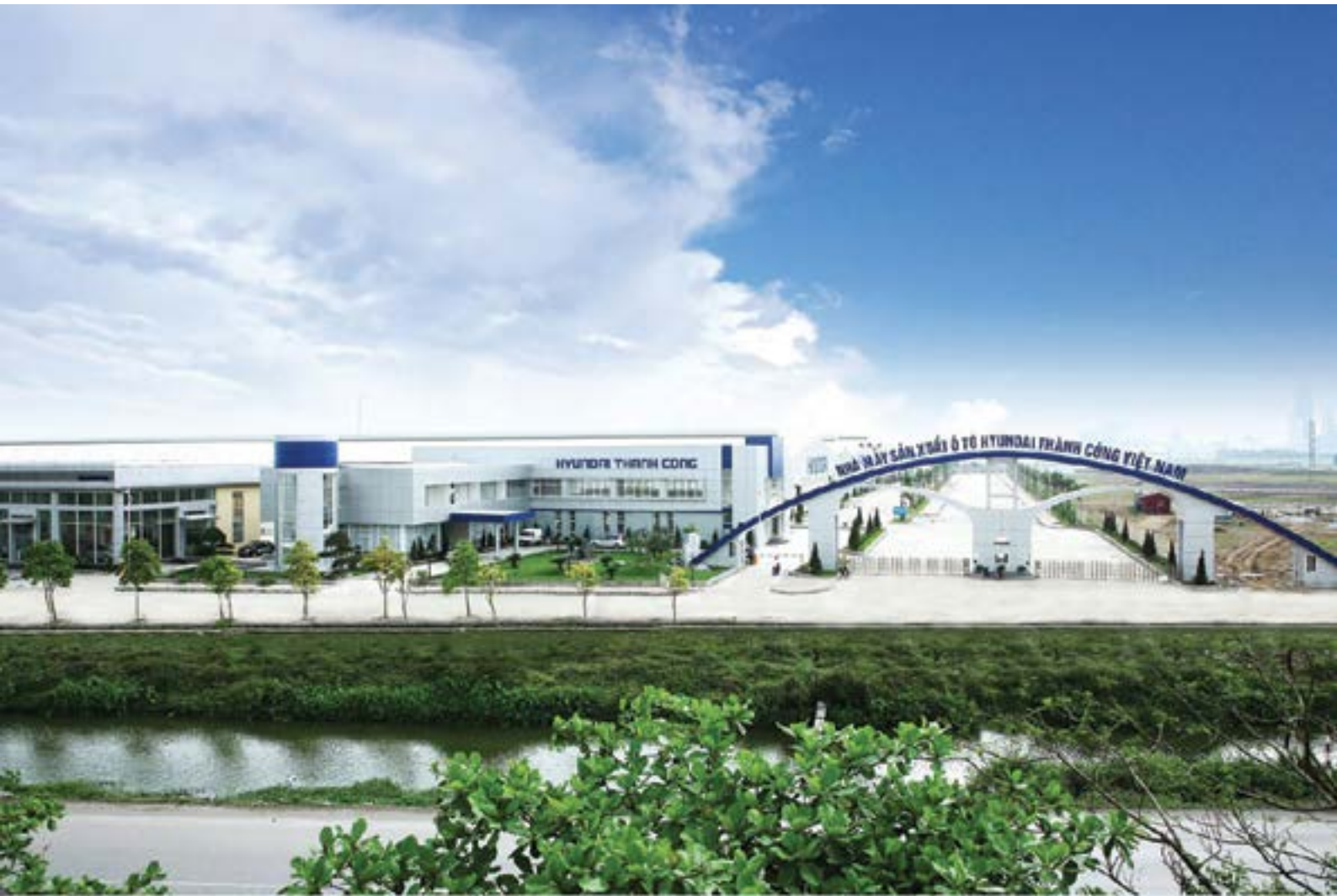
Hyundai Facilities, Ninh Binh, Vietnam
