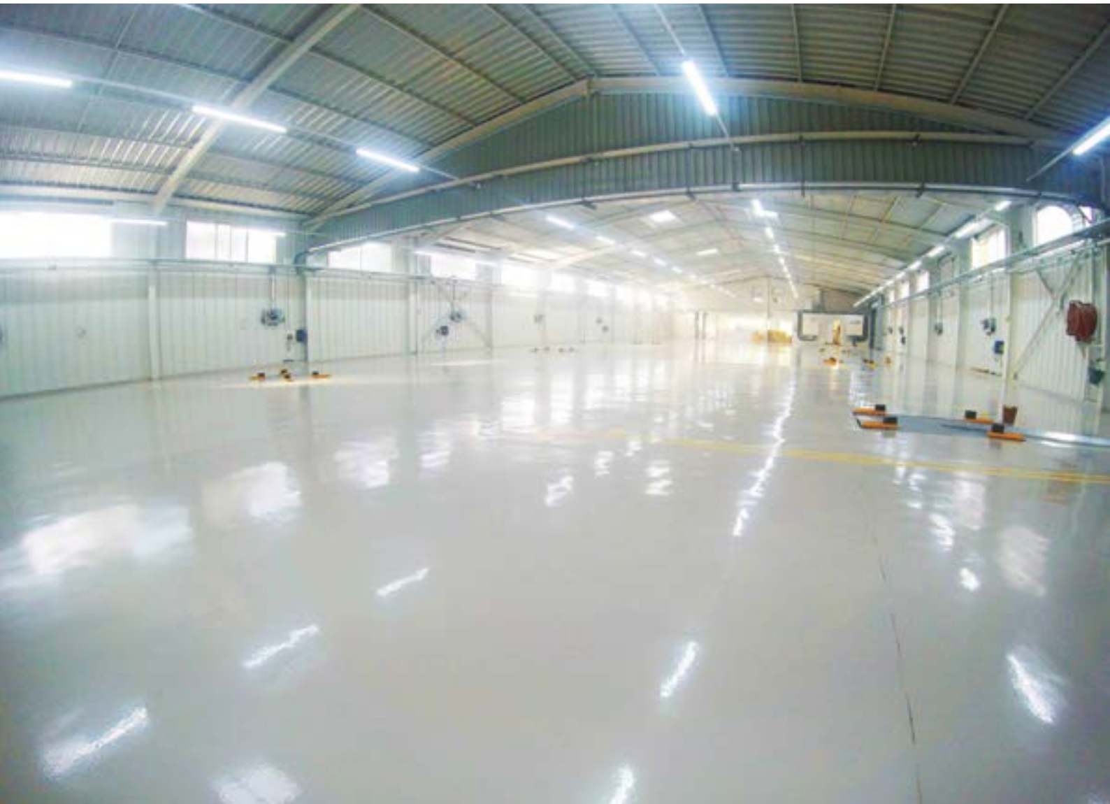
Preparation center for luxury vehicles, Côte d'Azur, France
